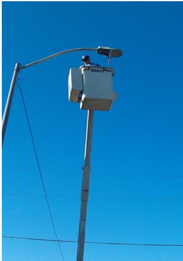
Andy Hubbard makes necessary repairs to a street light
